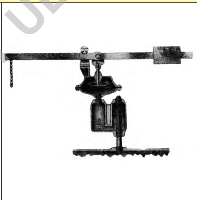
Fire governor with pocket and membrane (1930 Chappée Catalog *)
